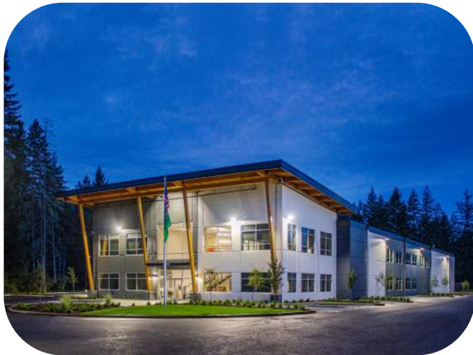
The new Carpenters Training Center at DuPont, WA.
