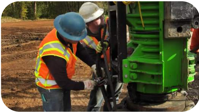
Piledrivers training with a diesel 'hammer' at Canby, WA.
